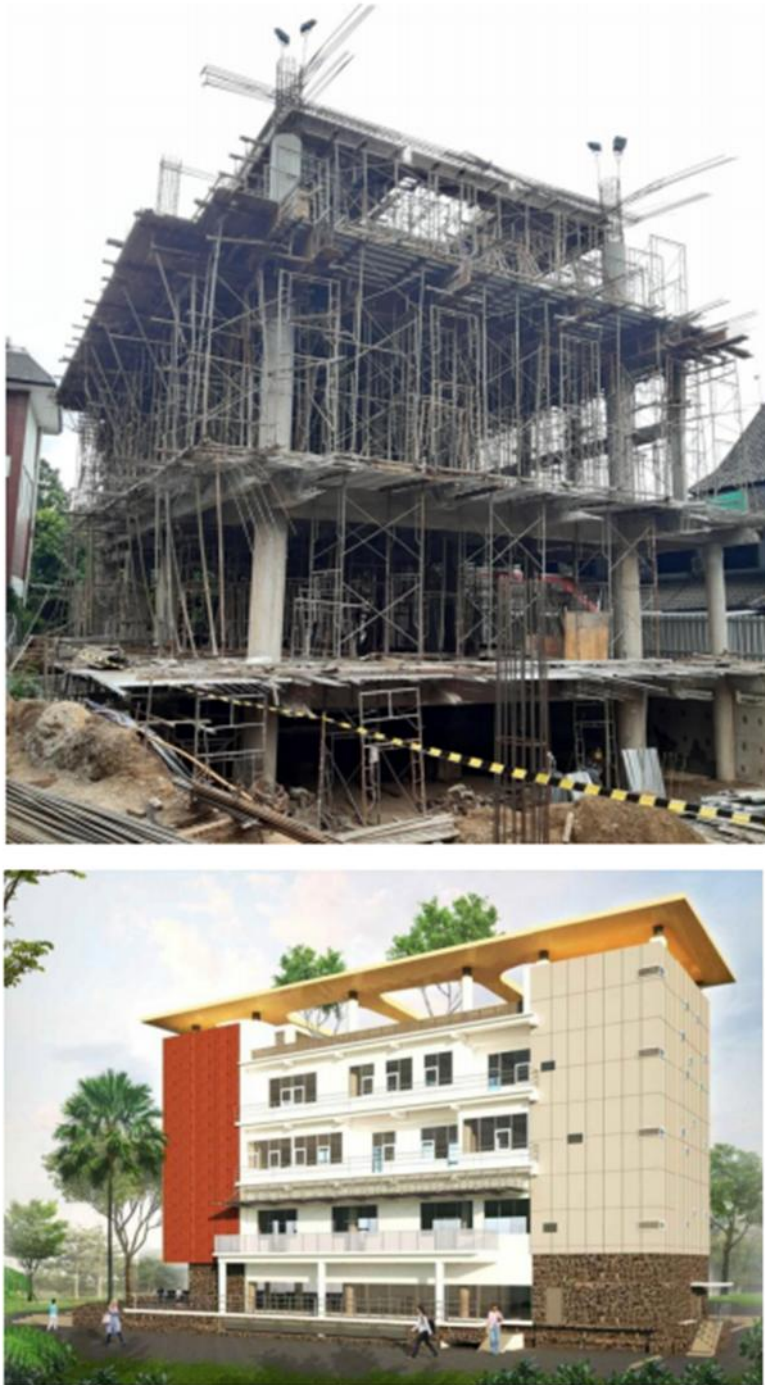
Gambar 3.18. Pembangunan Gedung Science and Techno Park (Atas) dan Gambar Detail Engineering Design Gedung Science and Techno Park (Bawah)
