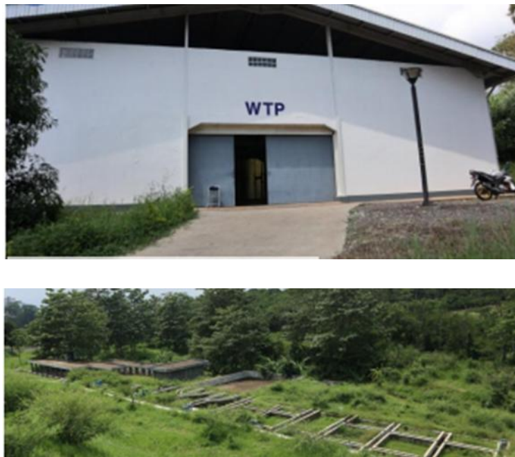
Gambar 3.24. Gedung Water Treatment Plant (Atas) dan Laboratorium Lapangan Air (Bawah)
